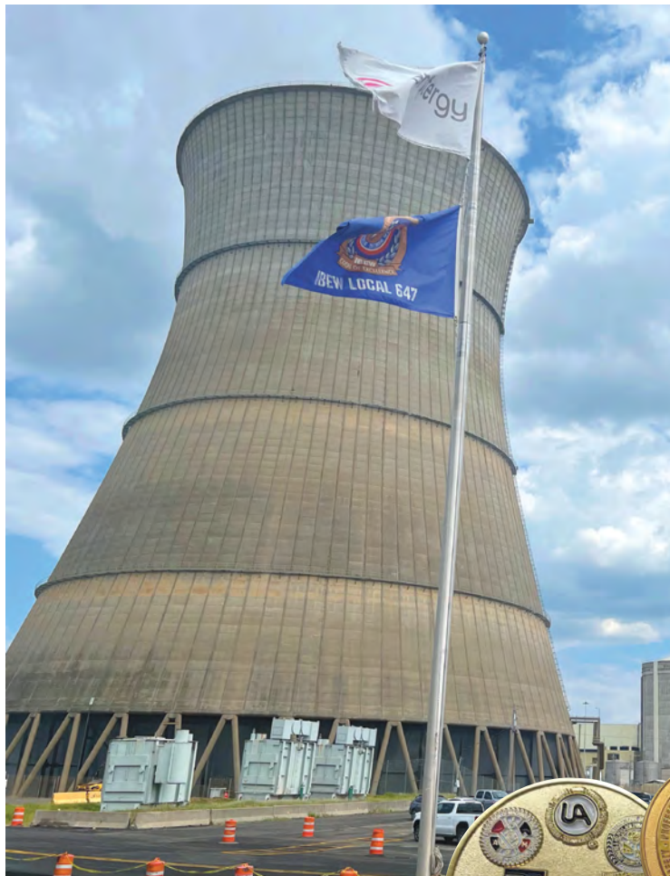
Little Rock Local 647's flag flies just below the corporate flag at the Enertgy Arkansas Nuclear One plant in Russellville, signifying a culture of respect and cooperation that helped save the plant from being shut down in the last decade.
